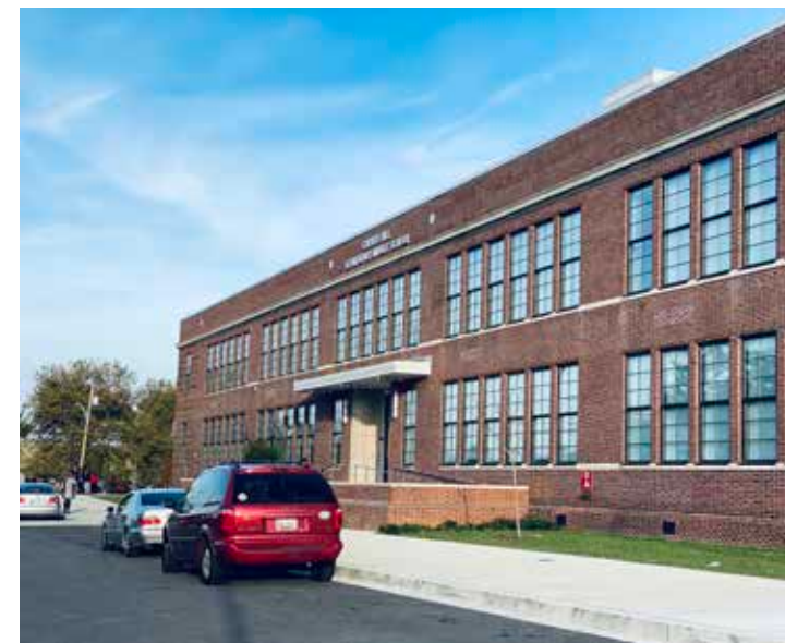
Newly Renovated portion of Cherry Hill Elementary/Middle School
