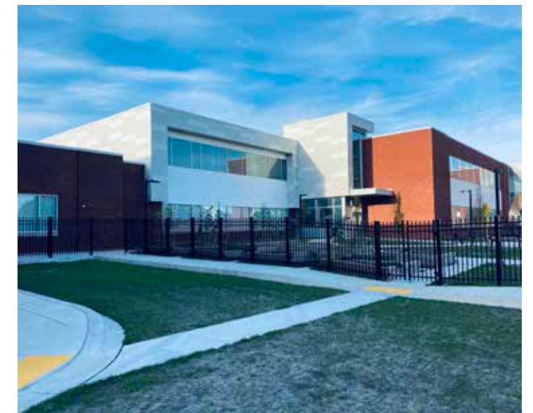
New addition and expansion of Cherry Hill Elementary/Middle School
