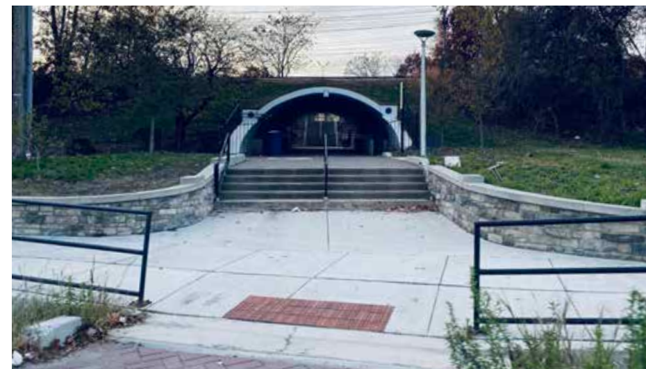
Existing tunnel connection to Cherry Hill Station
