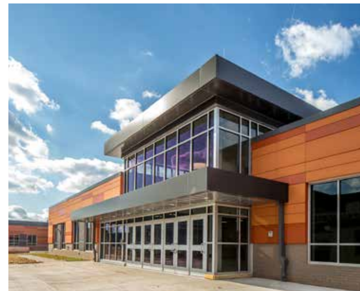
Newly constructed Arundel Elementary School
